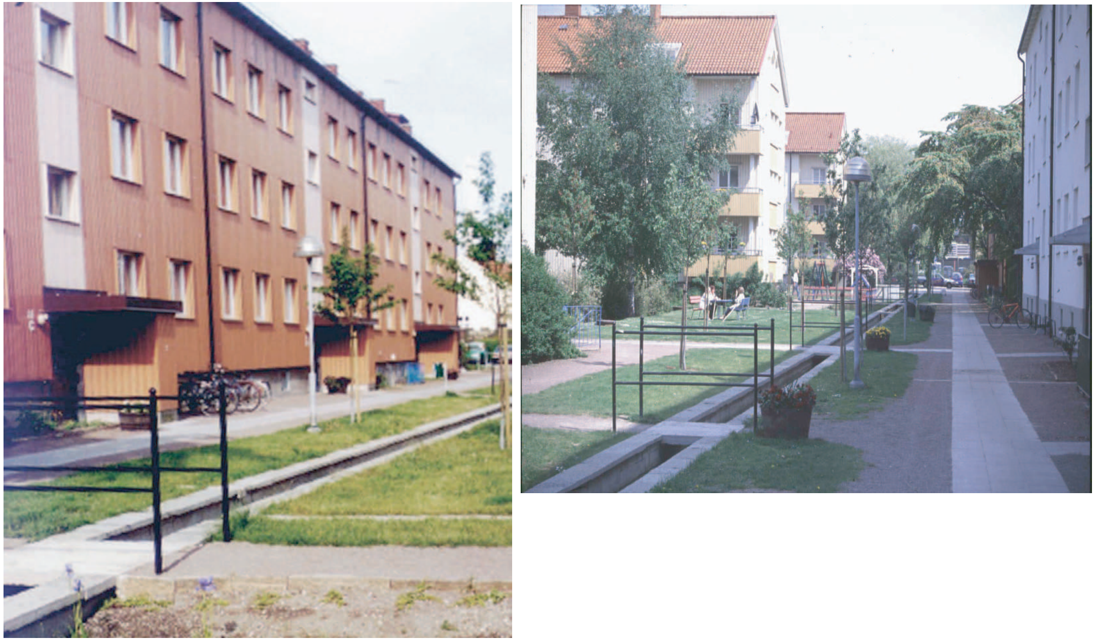
Change of previous insulation on the facades and local treatment of storm water Malmö
