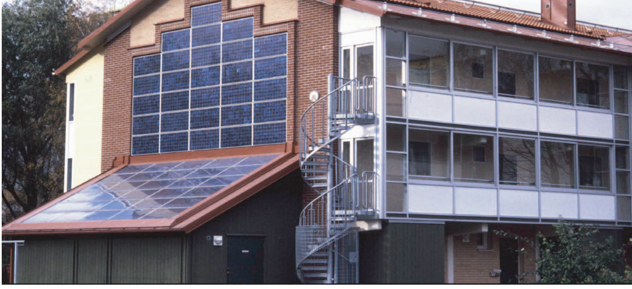
Addition of photovoltaic panels to the facade Kristianstad
